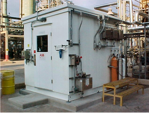
FHR BTX Heaters CEMS (4 Stack System) NO x , CO, O 2
