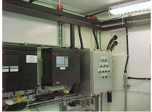
FHR BTX Heaters CEMS (4 Stack System) NO x , CO, O 2
